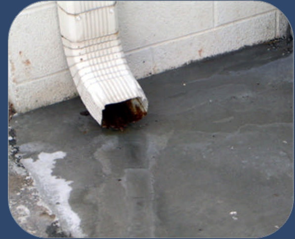
Misdirected roof drain
