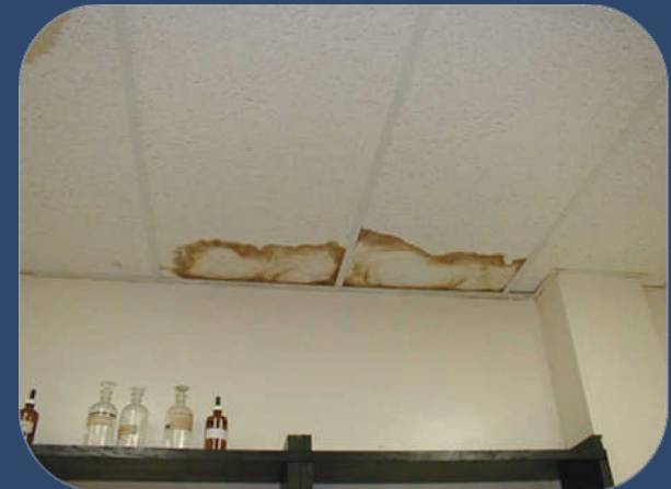
Water leak above ceiling
