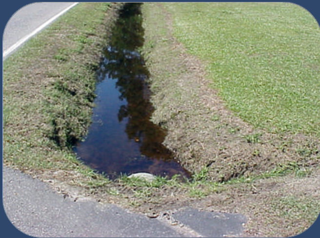
Clogged drainage ditch at school entrance
